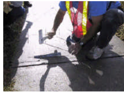
CRACK STITCHING: Galvanized steel blades being installed before Fusion-Crete® is applied.
